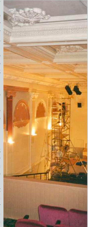
Detailed work on the auditorium arches.
