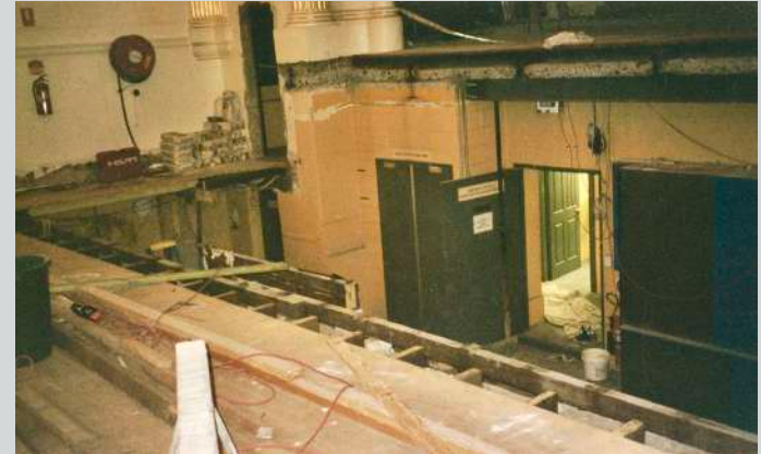
Work in preparation for the new raised pit.
